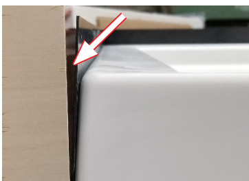
Screw flange to wall stud.
